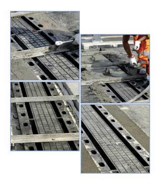
Expansion joints are installed on bridges to prevent interruption and to keep conjunction of bridge's surface. For keeping safety of bridge, expansion joints must have special features like; movement, high elasticity, resistance against impact, cold and hot weather.
